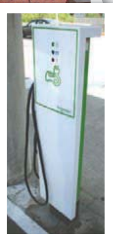
Charging station on roof of Discovery Place Deck: The charging station at Discovery Place is fueled by the electricity generated by the facility's photovoltaic system.
