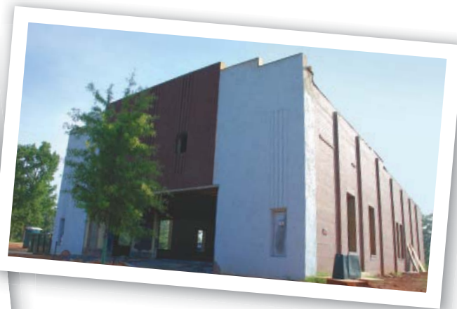
Belvedere Theater After: The building was completely re-purposed and retrofitted into an energy efficient dentist office with a white membrane roof that reflects sunlight, a tankless water system and high efficiency windows. Sub-recipient Dest Dental, received a $63,000 grant from the Commercial Building Retrofit Program. Dest paid for dental equipment, including X-ray machines. This project leveraged $1.5 Million of private funds from Dest Dental Management.
