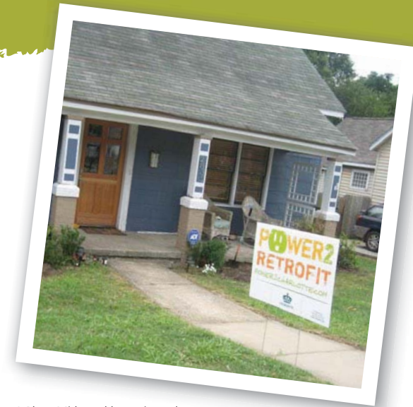
A Plaza-Midwood home is made more energy efficient thanks to an energy audit and repairs made as part of the Neighborhood Energy Challenge.
